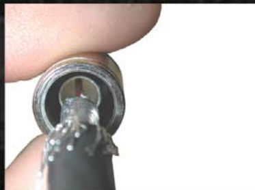
Guide center conductor and dielectric into post. Insert cable into connector until dielectric is flush with surface of post
